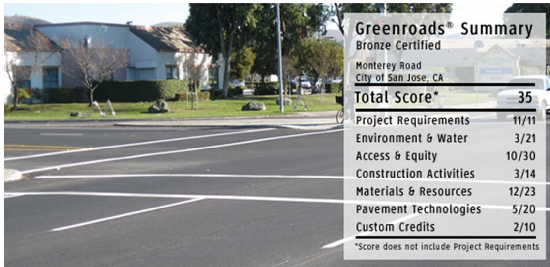
Monterey Road Reconstruction Project’s Greenroads Scorecard. The project completed all 11 Project Requirements and 14 credits worth 35 points, earning a Bronze Certification.
